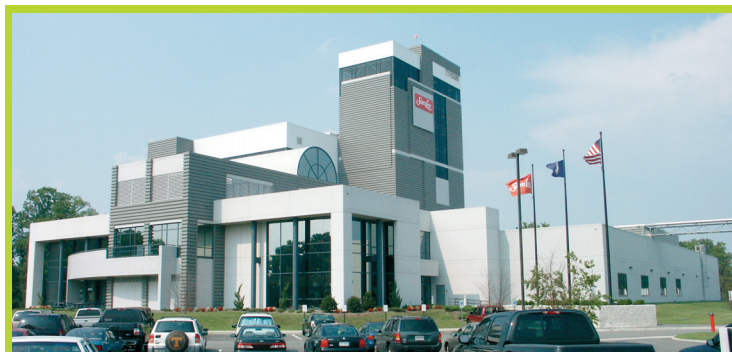
Sara Lee's Douwe Egberts coffee production plant in Suffolk, VA
